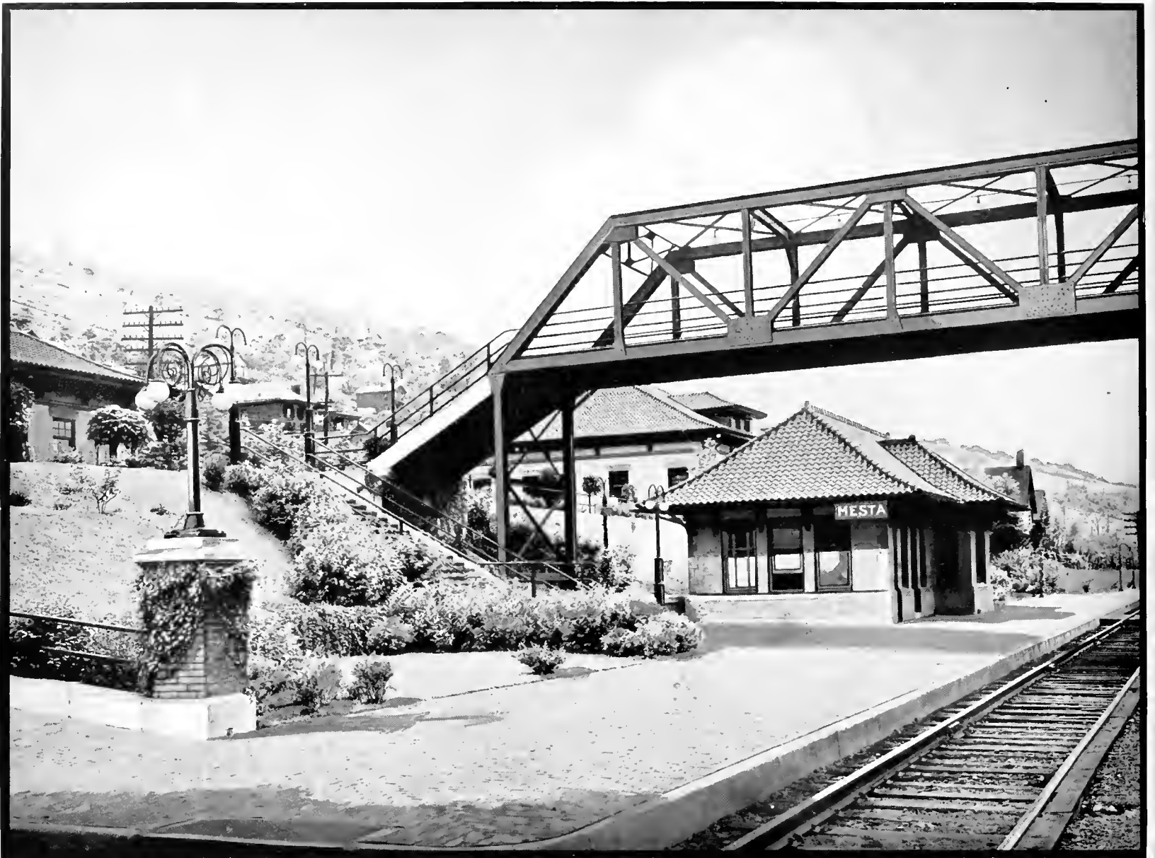
Mesta Station, Pennsylvania Railroad, West Homestead, Pa.
